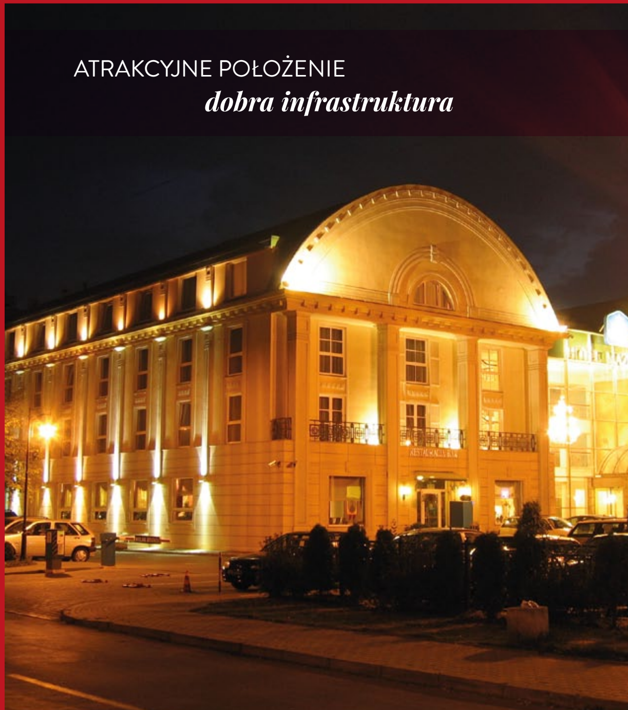
MCC Mazurkas Conference Centre & Hotel w Ożarowie Mazowieckim.
